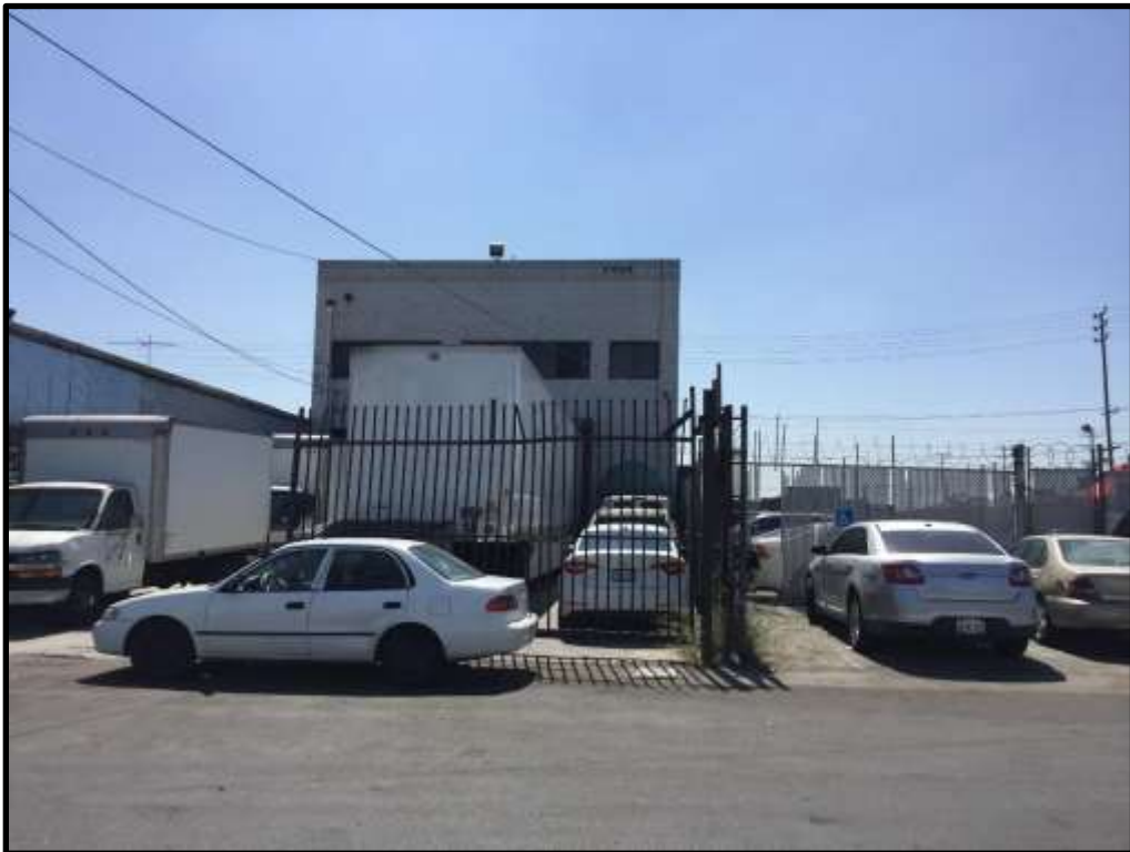
12. The northerly adjacent building and the Project Site, facing south from across Bay Street from the Project Site.
