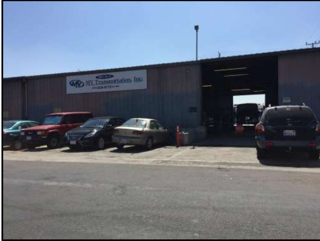
7. The Project Site, facing south from across Bay Street.
