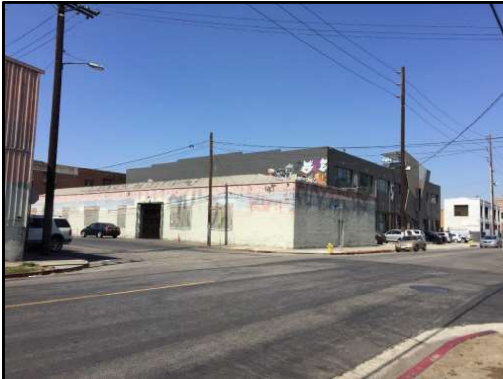
14. Caddy corner from the Project Site, facing northwest from the southeast corner of the intersection of Bay Street and Mateo Street.
